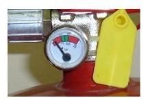
Check the pressure reading on the gauge.
