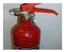
No pressure means the unit will not function. Over-pressure could result in a failure of the seals. Check the condition of equipment for missing or damaged pieces.
