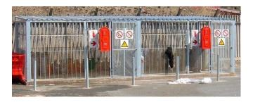
For ease of management, different gasses are to be separated from each other and empty cylinders marked "MT"
