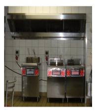
Extraction hoods are to be installed over the deep fat fryers. The filters are to be cleaned daily and the flue pipes every 3 to 6 months. A cleaning certificate is to be obtained from the Cleaning Company.
