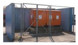
To prevent malicious interference, transformers should be housed in a secured location or fenced off. Oil cooled transformers need to have bund walls to contain any spillage. The **silica gel** should always be **blue** in colour. The changing to pink indicates that moisture is no longer being effectively absorbed from out of the oil. The result that the oil can breakdown, start to heat up and could result in a fire within the transformer.
